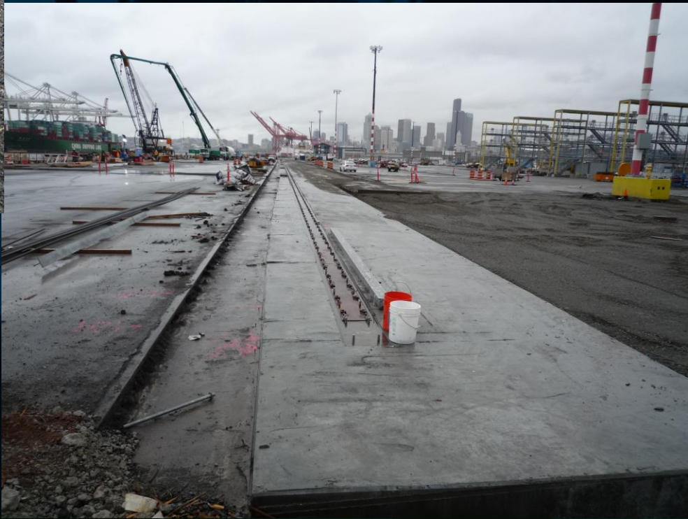
Landside Crane Beam work February 2009
