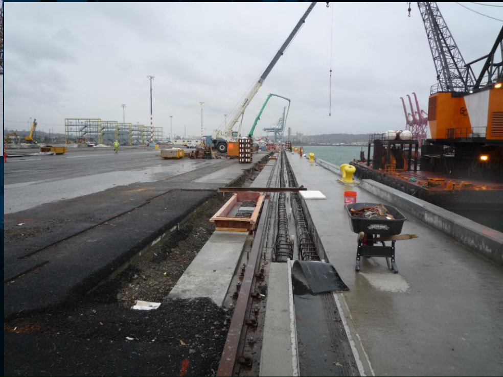
Waterside Crane Beam work February 2009
